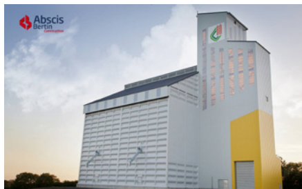
Silo Sept Vents
