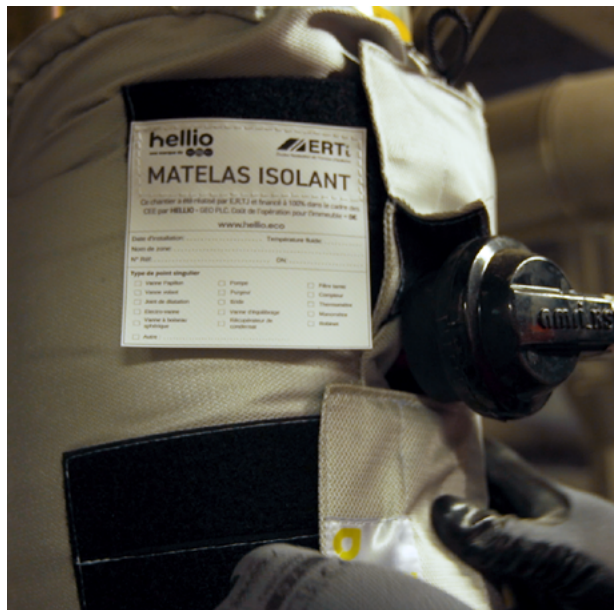
Matelas isolant - © photo HELLIO
