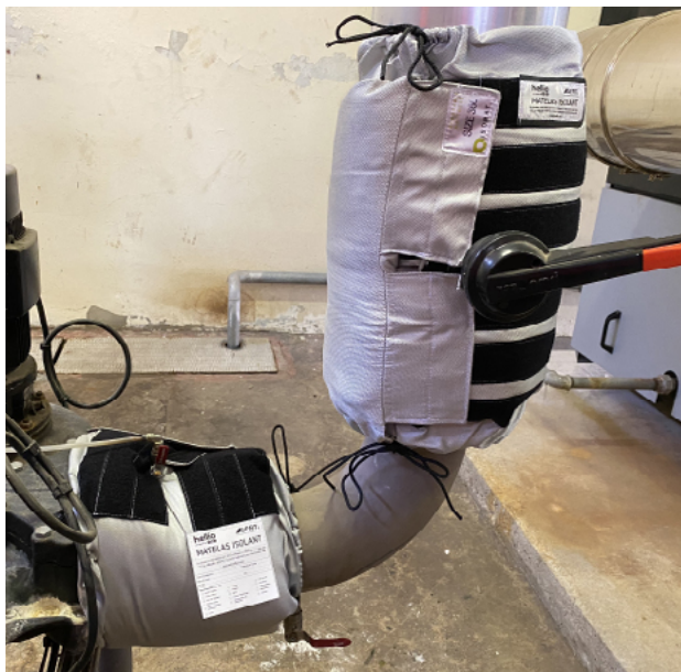
Isolation des points singuliers - © photo HELLIO
