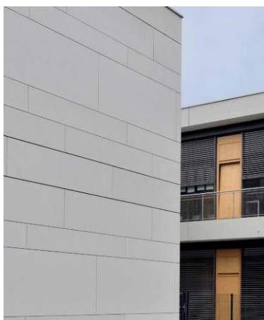
American International School à Zagreb StoVentec FibreCement
