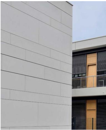
American International School à Zagreb StoVentec FibreCement
