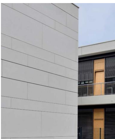
American International School à Zagreb StoVentec FibreCement
